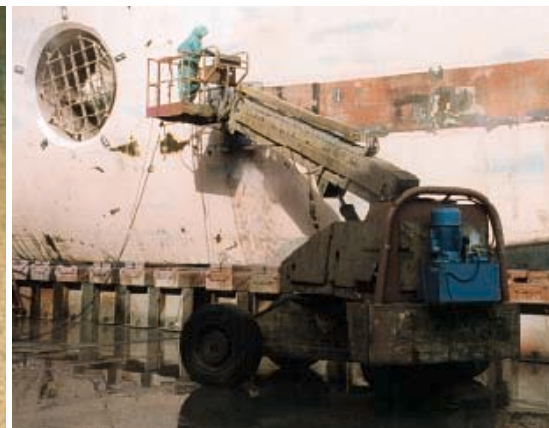
Surface preparation for corrosion protection
