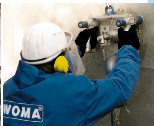
Decoating of concrete surfaces
