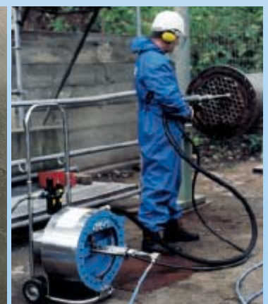
Cleaning of tube bundles with simultaneous waste recovery
